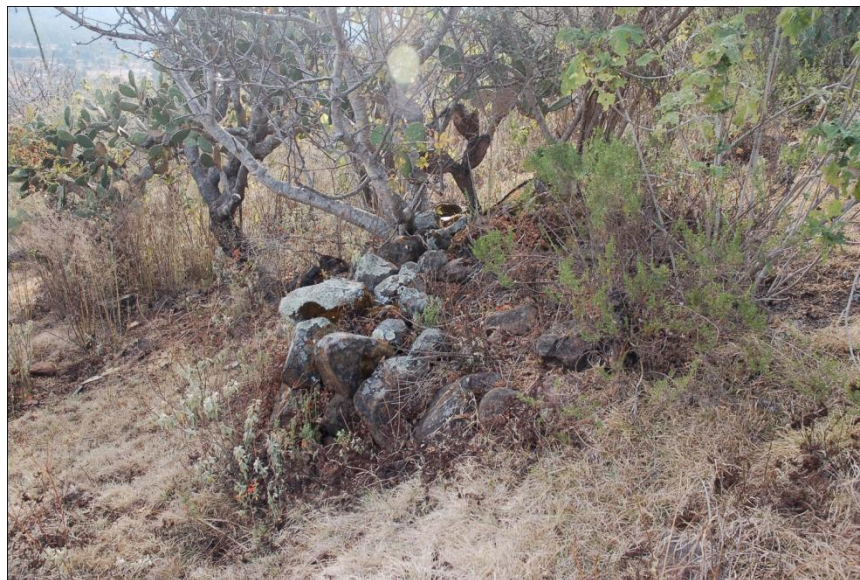
Fig. 6.17. Type C Terraces (structure 11 incorporated into the terrace as retaining wall)
