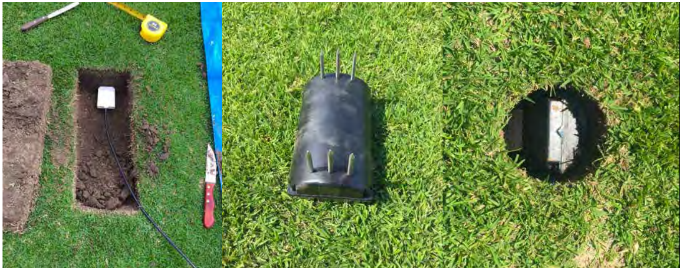
Figure 2. Campbell Scientific (CS655, left panel) and Toro Turf Guard (right two panels) soil moisture sensors were installed in each plot. Photos by Don (Wes) Dyer.
