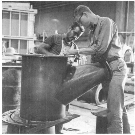
Fig. 6(b) Fitting a branch connection
