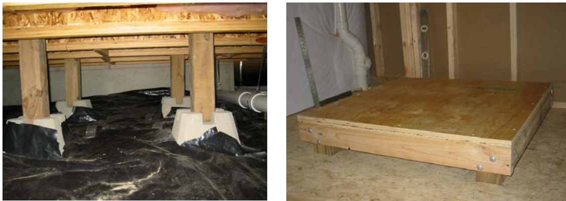
Figure B-5: Tank support platform
