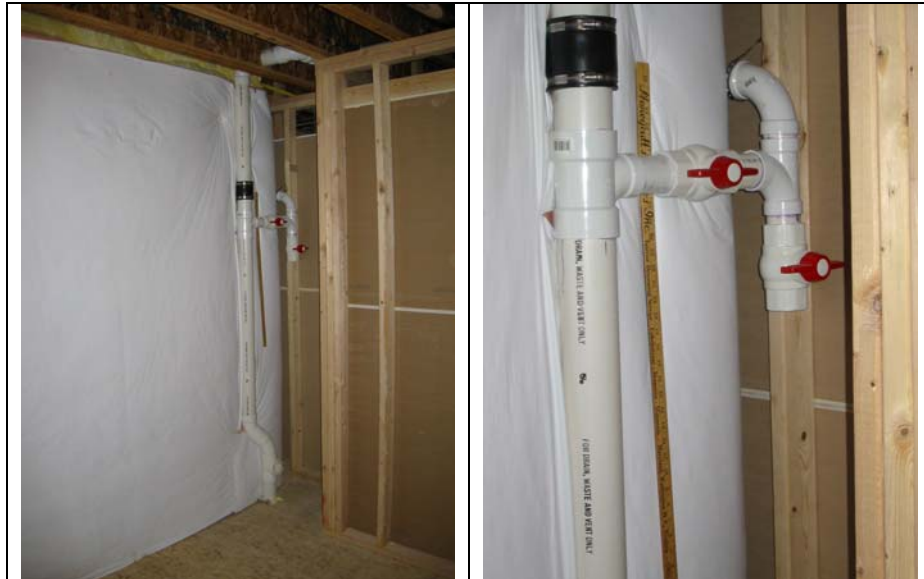
Figure B-1: Residential graywater system connection point
