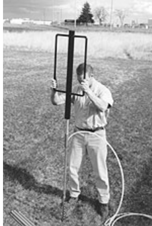
Figure 3-2 Driving Piezometers with a Slide Hammer
