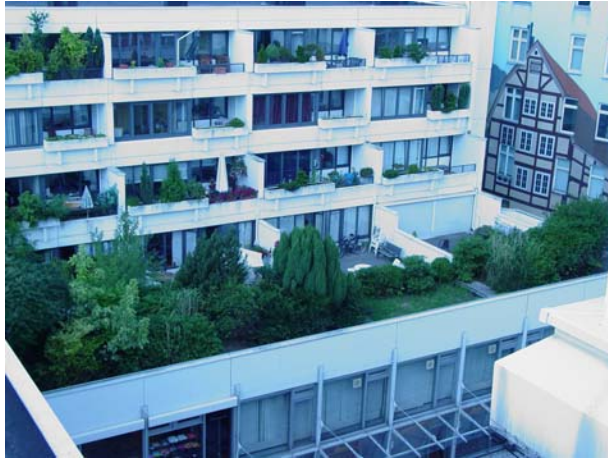
Figure 4.25 Poeseldorf Apartments. Intensive green roofs provide cooling benefits for shops below and aesthetics for the apartments above.
