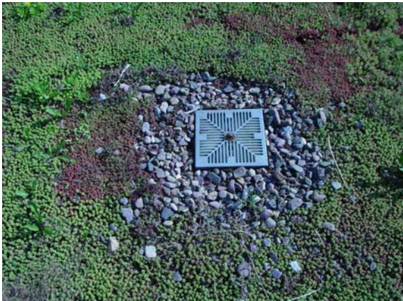
Figure 4.11 Green Roof Drain. Gravel around drain facilitates drainage. Sedums are beginning to creep into the gravel area.
