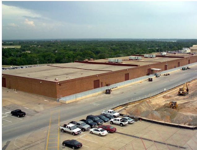
Figure 4.1 Building 15 at AFP 4 in Ft. Worth, TX. Building 15 has over 100,000 ft 2 of roof. (Rowls, 2003)
