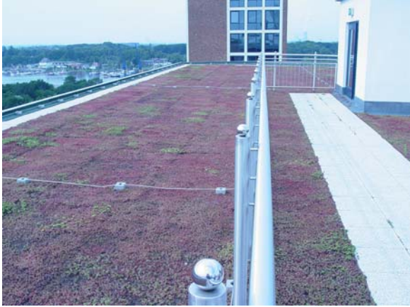
Figure 4.27 WIRO GmbH Roof. Facility occupants take work breaks on this extensive green roof.
