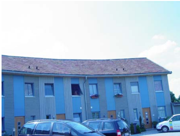
Figure 4.23 Apartment Building. The vegetation on the 2 year old apartment building was installed as vegetated mats.
