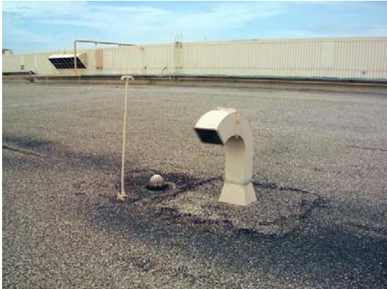
Figure 2.1 Asphalt BUR. Roof drain and vent.
