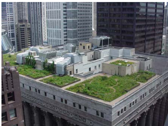
Figure 4.2 Chicago City Hall Green Roof. Note the black roof on the county's portion of the building in the back right.
