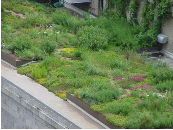
Figure 4.4 City Hall Roof. Note the variety of plant species on the roof as well as the extensive versus the deeper semi-intensive sections of the roof.
