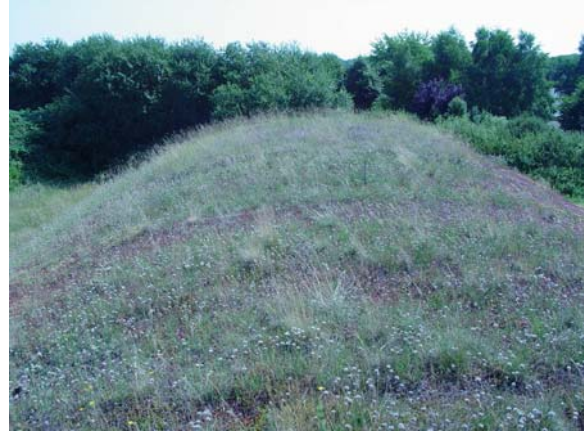
Figure 4.14 Bunker 1. The top of the bunker is flat enough that soil can remain in place.
