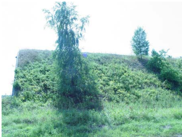
Figure 4.17 Bunker 2. With soil depths ranging from 20 cm to 1 meter, the intensive roof on bunker 2 is able to sustain large trees as well as other vegetation.
