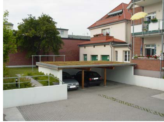
Figure 4.30 Green Roof Carport. Green roof over a carport – reducing storm water runoff.
