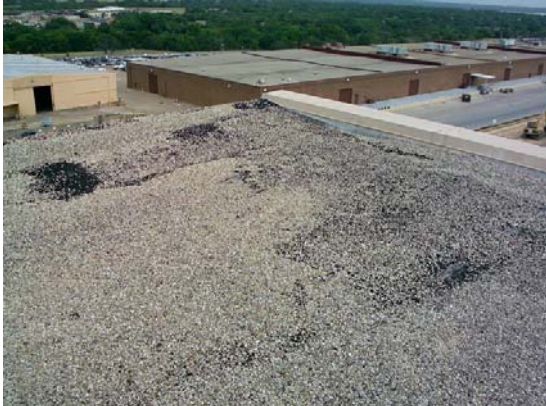
Figure 2.2 Asphalt BUR. Corner of Asphalt BUR and Building 15 in background.
