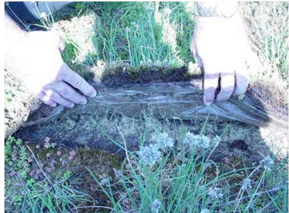
Figure 4.12 Green Roof Mats. No growing medium was used on this roof except the substrate in which the mats were grown before installation.
