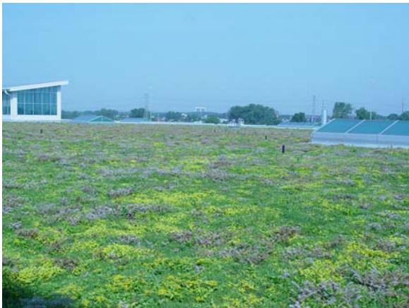
Figure 4.7 Ford Roof. The Ford River Rouge truck manufacturing plant roof is currently the largest green roof in the world. A light monitor (seen in background) allows natural light into the plant.
