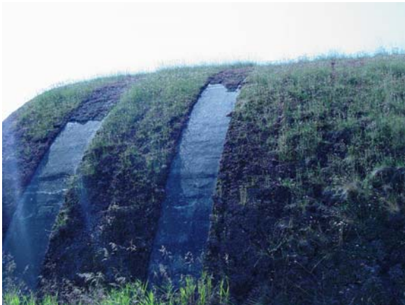
Figure 4.15 Bunker 1. The steep sides of the bunkers are not as conducive for plant growth without additional mechanisms to support a growing medium.
