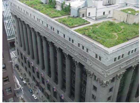
Figure 4.5 City Hall Roof. Chicago City Hall is approximately 8 stories above the street level. Materials were placed on the roof by crane and freight elevator.
