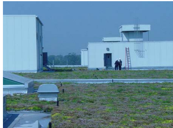
Figure 4.8 Ford Roof. Workers from the installation contractor maintained the roof for one year after installation (Russell, 2003).
