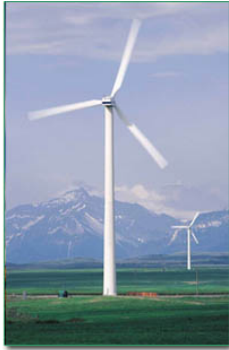
Figure 2. A Horizontal-axis Three-bladed Turbine (Vision Quest Windelectric, 2003)
