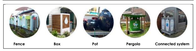
Figure 7.18 Types of small-scale rainwater storage (Source: SG, 2018)
