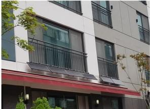
**Figure 8.1** Small-scale solar energy generator installed on the veranda rail in two rows (left) and between floors (right)
