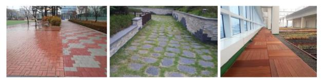
Figure 7.19 Permeable pavements (blocks) in Jangan district office (Source: SG, 2014)
