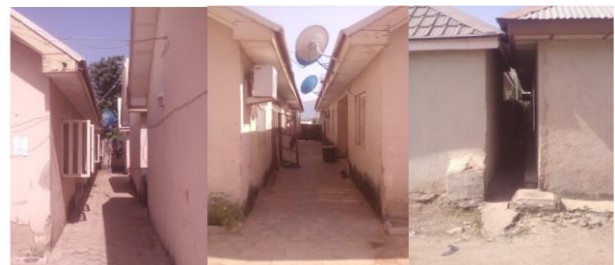
Figure 3. Windows of houses opening into a narrow lobby with insufficient setbacks between buildings, causing insufficient airflow for adequate ventilation.
