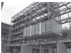
Fig 7. Module with corner and intermediate posts supported by a structural frame, courtesy of Yorkon and Jule engineers.
