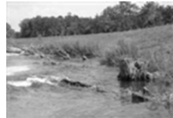
Riffle-pool bypass channel on the Traisen river, St. Poelten, Austria. Picture Source: [10]
