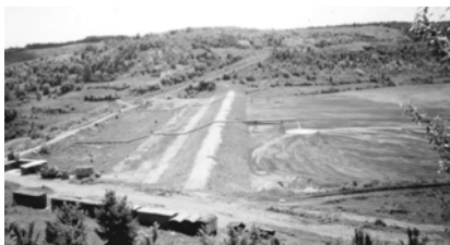
Figure no. 2. Ceplea Valley deposit of Energy Complex Turceni
