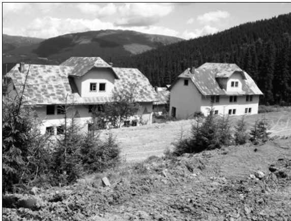
Photo: Social Fiches in Calimani Mt, 1550m alt., former buildings for service
