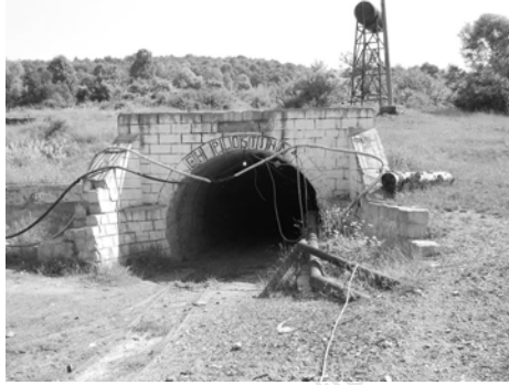
Figure 3 Entry in coal mine (Riti, 2011)
