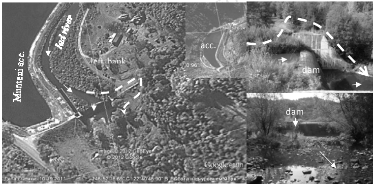
Figure 11. Possible location of the bypass channel (Picture Source: Google earth, 2011 (left) E.Luca (right))
