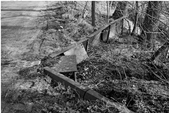
Figure 2. Tunnels for amphibians
