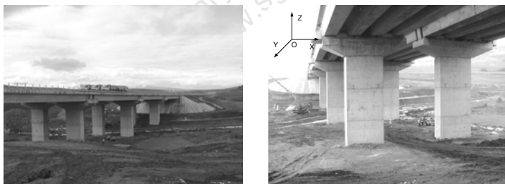
Fig. 1 The bridge deck
