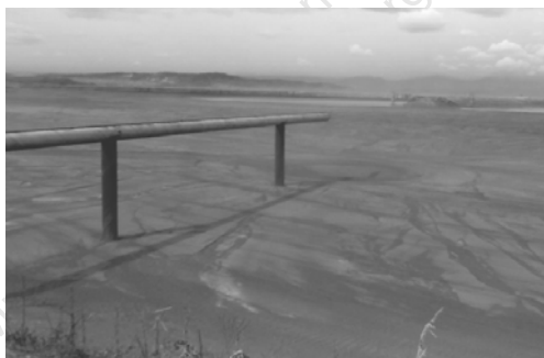
Fig. 1. Ash and slag storehouse from Valea Ceplea – Turceni
