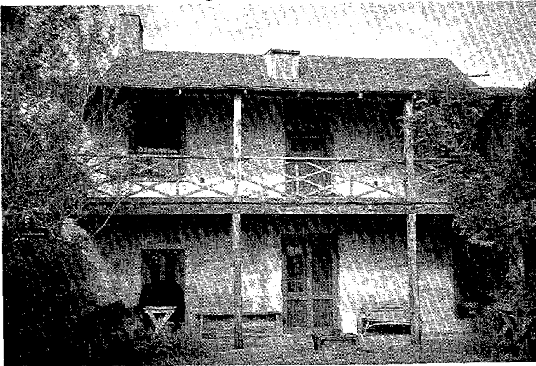
19B Garden Facade, Long-Sánchez House
