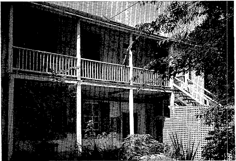
24B Garden Facade, Poujoud-Slater House
