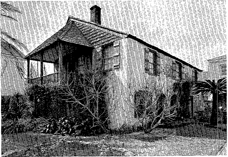
12A Garden Facade, Oldest House
