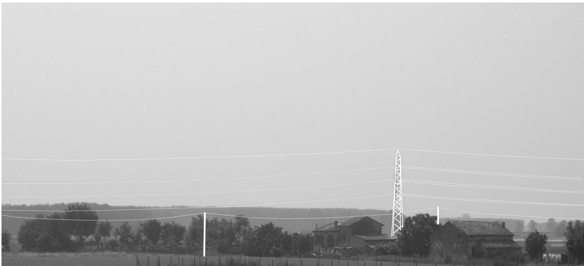
Figure 3.7 The direct layer of a transmission line as underlined by landscape architects in the analysis of the landscape perception, Guastalla, Emilia Romagna. In this case the line afflict the quality of the perception. (image of the author, 2006).
