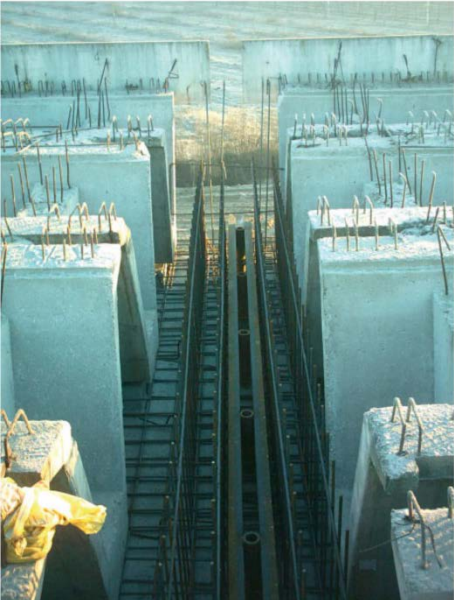
(c) Install steel beams and position rebar
