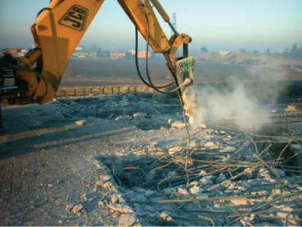
(a) Demolish concrete surfaces of slabs and girders
