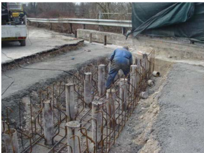
(a) Drill micro-piers
