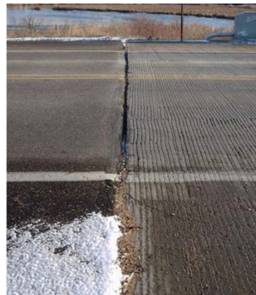
(b) Approach slab-pavement joint
