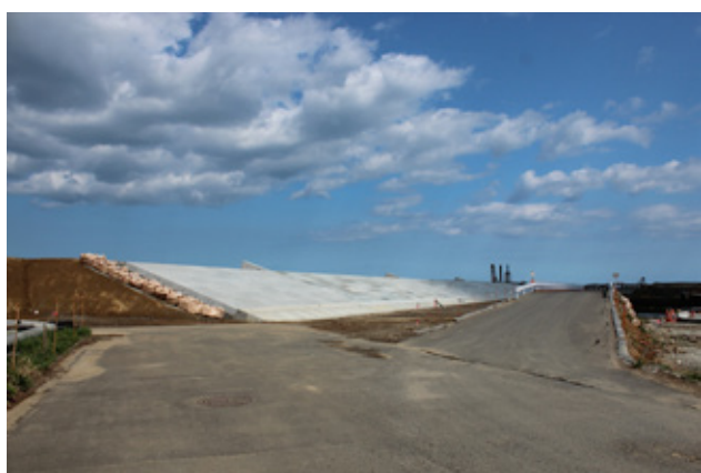
Fig. 4.19 Seawall Under Construction in Natori City
