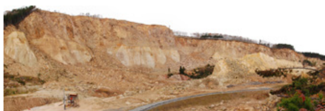
Fig. 2.10 Arato-zawa landslide area. The GB-SAR system can be seen at the bottom left
