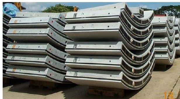
*Figure 9(b) Precast concrete segment lining*
