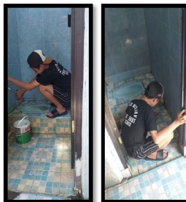
Gambar 7. Proses rehabilitasi minor lantai WC umum
