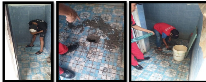
Gambar 1. Rehabilitasi minor system septik tank
