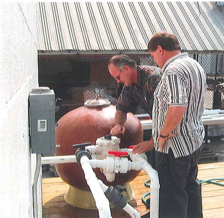
The pump which pulls water from the creek and pushes it through the sand filter
