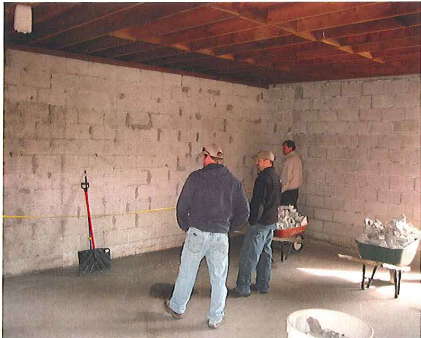
A storage room was stripped to the bare walls and refurbished
