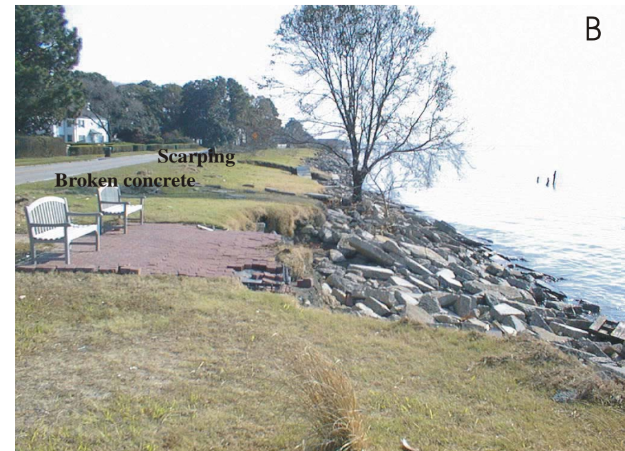
Figure 7. Hampton Roads shoreline after Hurricane Isabel A) at dune site Hp2 and B) along a typical shoreline. Photo date: 22 Sep 2003.
