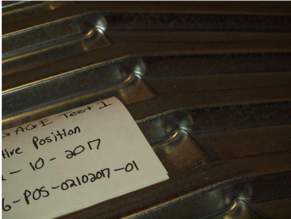
Figure 33: 16 Gage Deck Positive Bending – Both Ribs and Webs Buckling.
