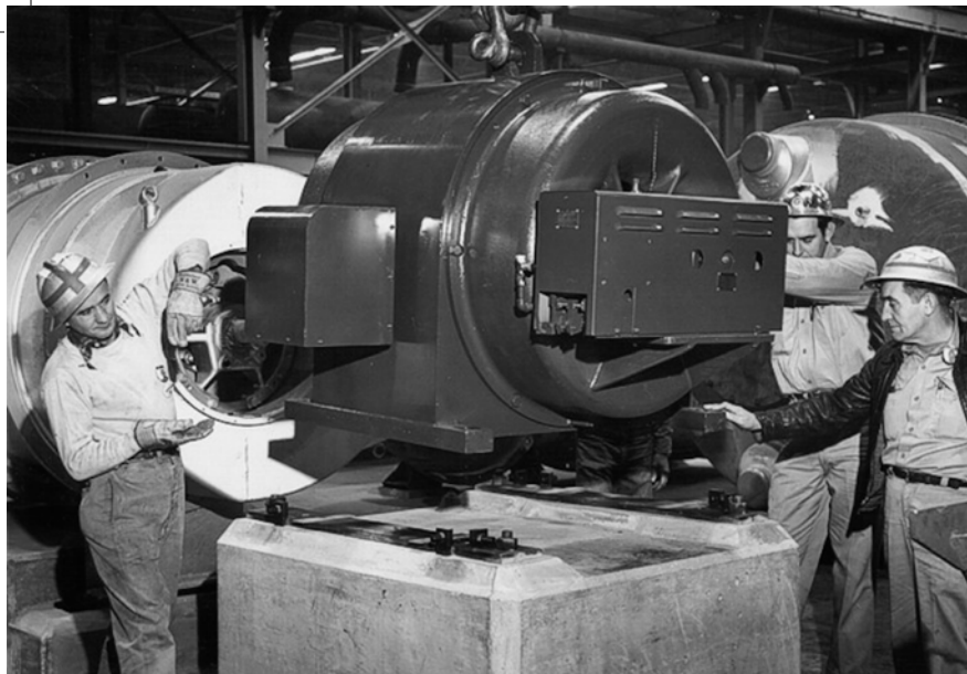
LEFT | In 1953, the X-330 Process Building installed its first compressor motor. Two years later, the Atomic Energy Commission acquired the process buildings.
