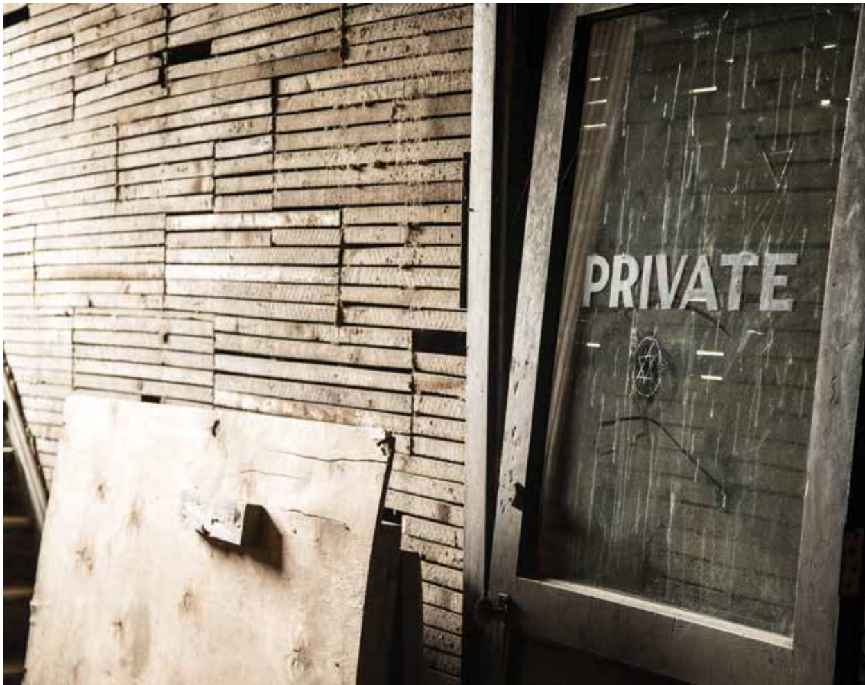
ABOVE | The Tecumseh Theater is three stories high and renovations are underway. The total cost of the project will be about $1.2 million.
