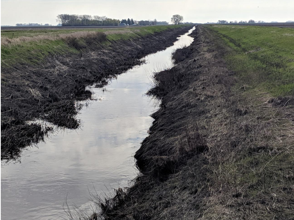
Figure 1. Drainage ditch in HIGDEM Township, Polk County, MN, on May 13, 2019 (Photo taken by the Author).
