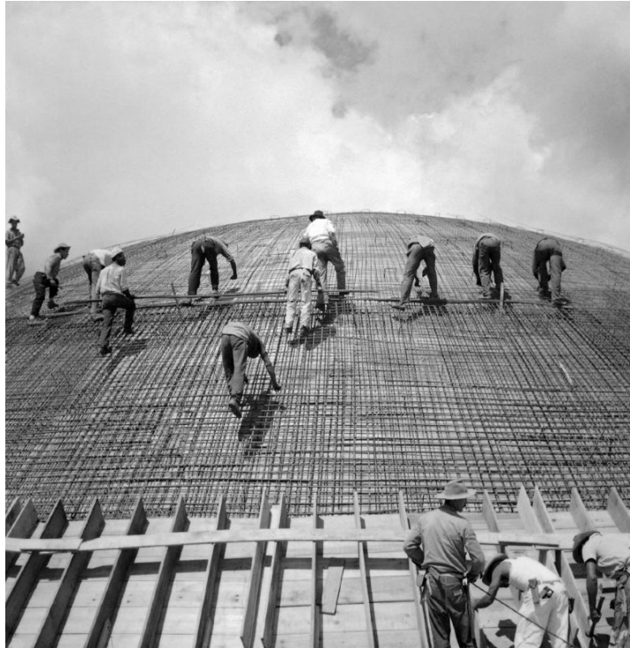
Figure 6.2 Marcel Gautherot. Construction of dome in Brasilia. 1959. (Source: Photo Instituto Moreira Salles.)
