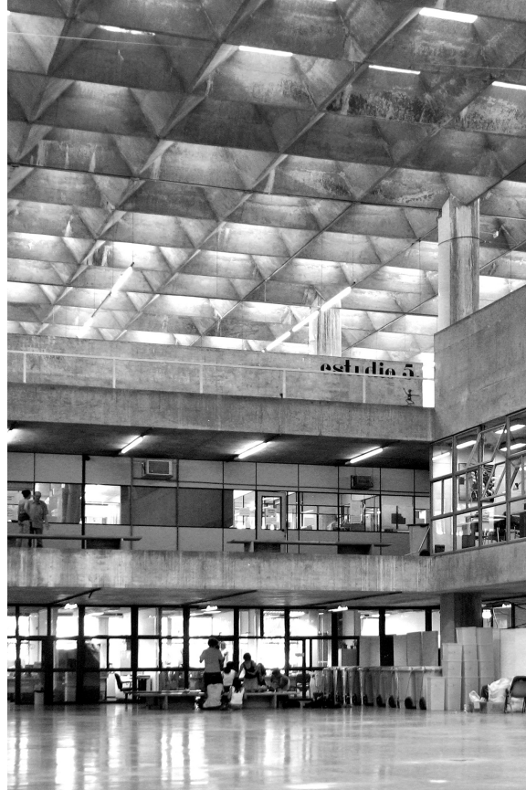
Figure 6.8 Central hall of FAU-USP.
