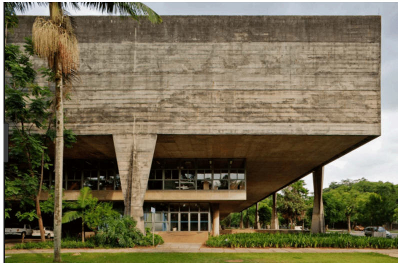
Figure 6.7 João Vilanova Artigas, School of Architecture and Urbanism of the University of São Paulo (FAU-USP), 1969.
