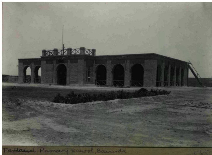
Figure 4.1 A view of Ferdowsi School, a model elementary school designed and built by the Company in Bawarda, circa 1931. Classrooms were organized around a central courtyard and were surrounded by an arched verandah.
