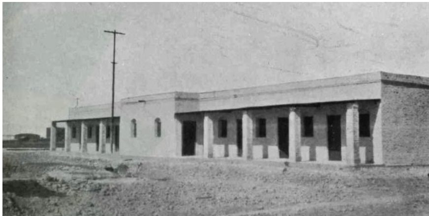
Figure 4.22 New Single Clerks' block under construction, October 1924. Each block consisted of eight rooms and two dining rooms, accommodating 8 men. Each room featured two windows and one door opening onto a verandah.
