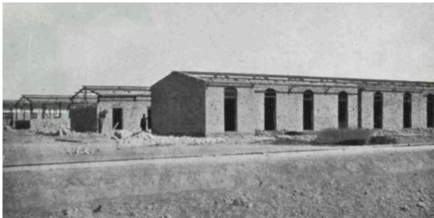
Figure 4.17 Artisans’ Single Quarters under construction, October 1924. Artisans were provided with the minimum level of housing standards. Each block was divided into ten rooms measuring 10 feet by 20 feet and featured a door on one side and a window on the other side, and no verandahs were provided.
