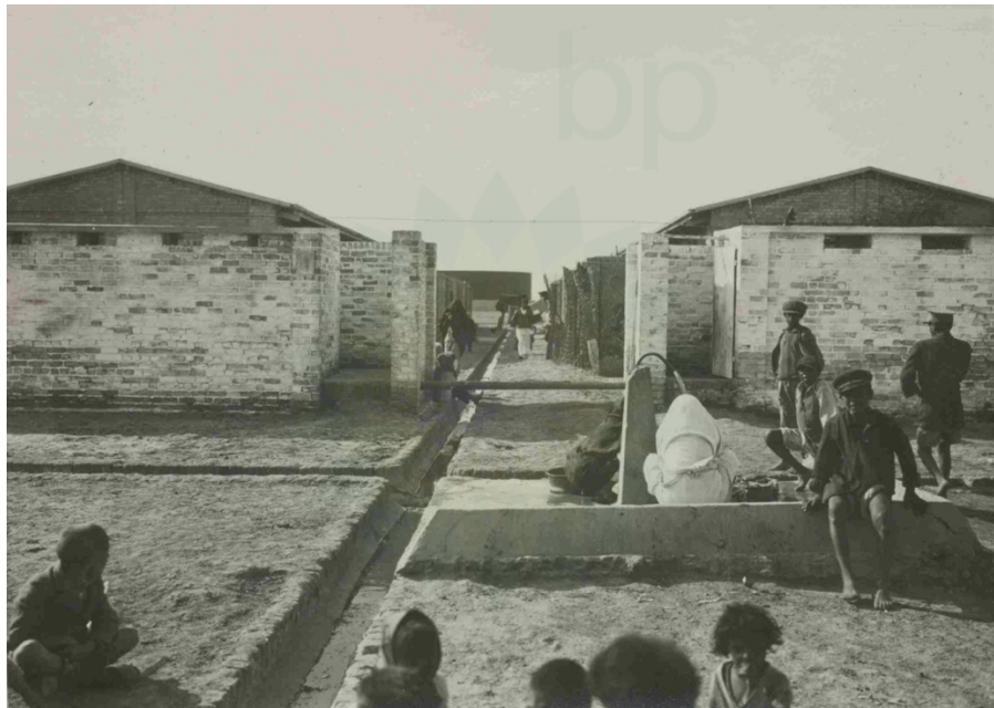
Figure 4.19 A view of Artisans' Married Quarters in the New Workmen's Village, circa 1935. Public water fountains were provided at regular intervals along the back-service alleys. Water fountains became social hotspots as they were frequented by housewives and children during the day. Source: BP Archives, ArcRef 229351
