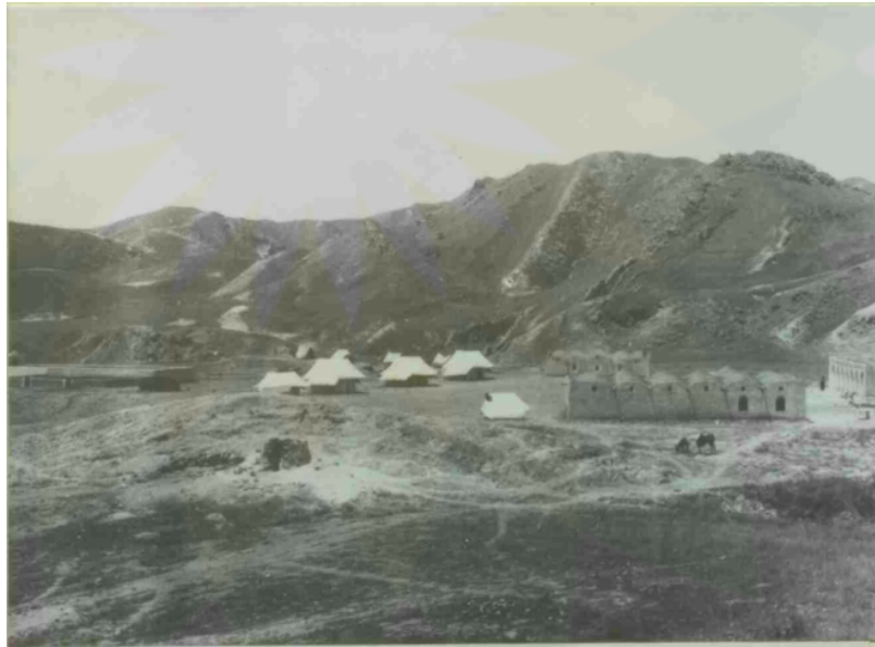
Figure 3.4 A photo of the first settlement in the Oil Fields, circa 1908. The caption reads: “Building on right with verandah was messroom and two bedrooms, building nearest camera was offices and that farthest from camera (near hills) was servants’ quarters.” Source: BP Archives, ArcRef 64874
