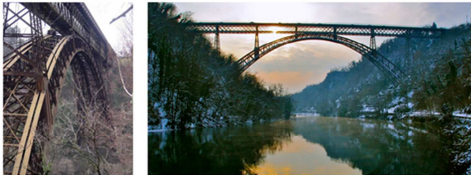
Fig. 1 Views of the San Michele iron arch bridge (1889). 41x15mm (300 x 300 DPI)
