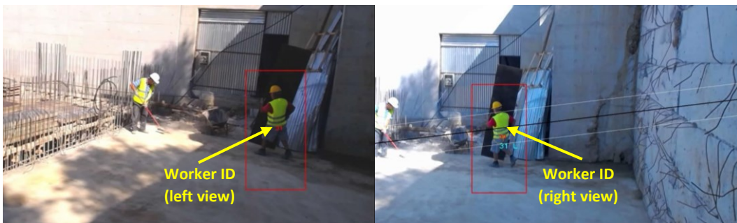
Figure 5. One worker ID matching across stereo frames.
