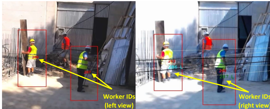
Figure 6. Two worker IDs matching across stereo frames.
