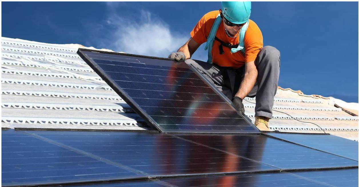
Figure 18: Fixing solar panels on the roof of the houses
