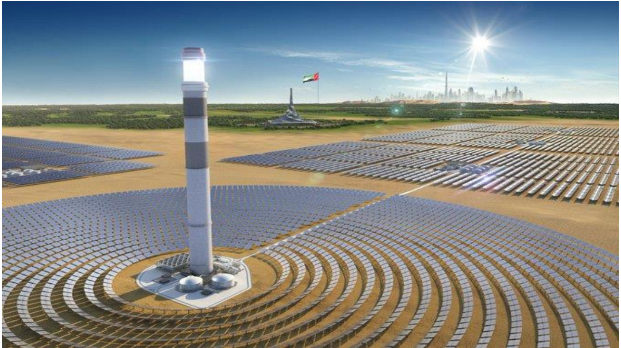
Figure 20: World's biggest Concentrated Solar Power project in Dubai
