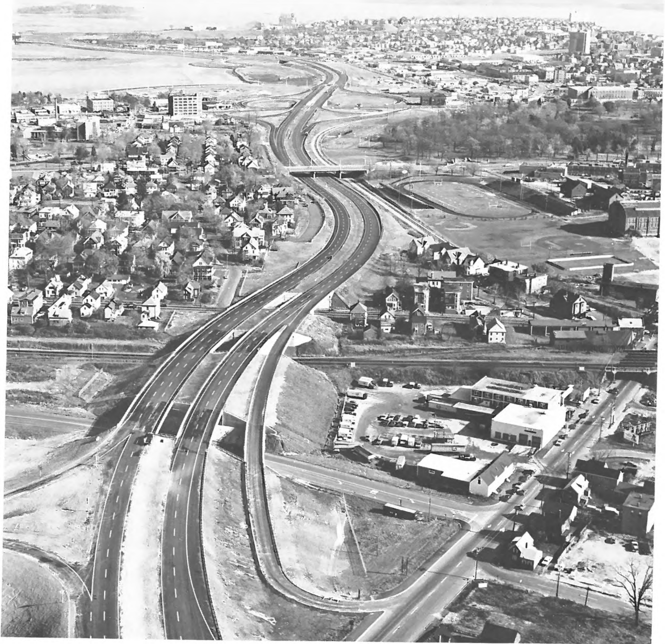
New section of I-295 expressway in Portland-South Portland.
