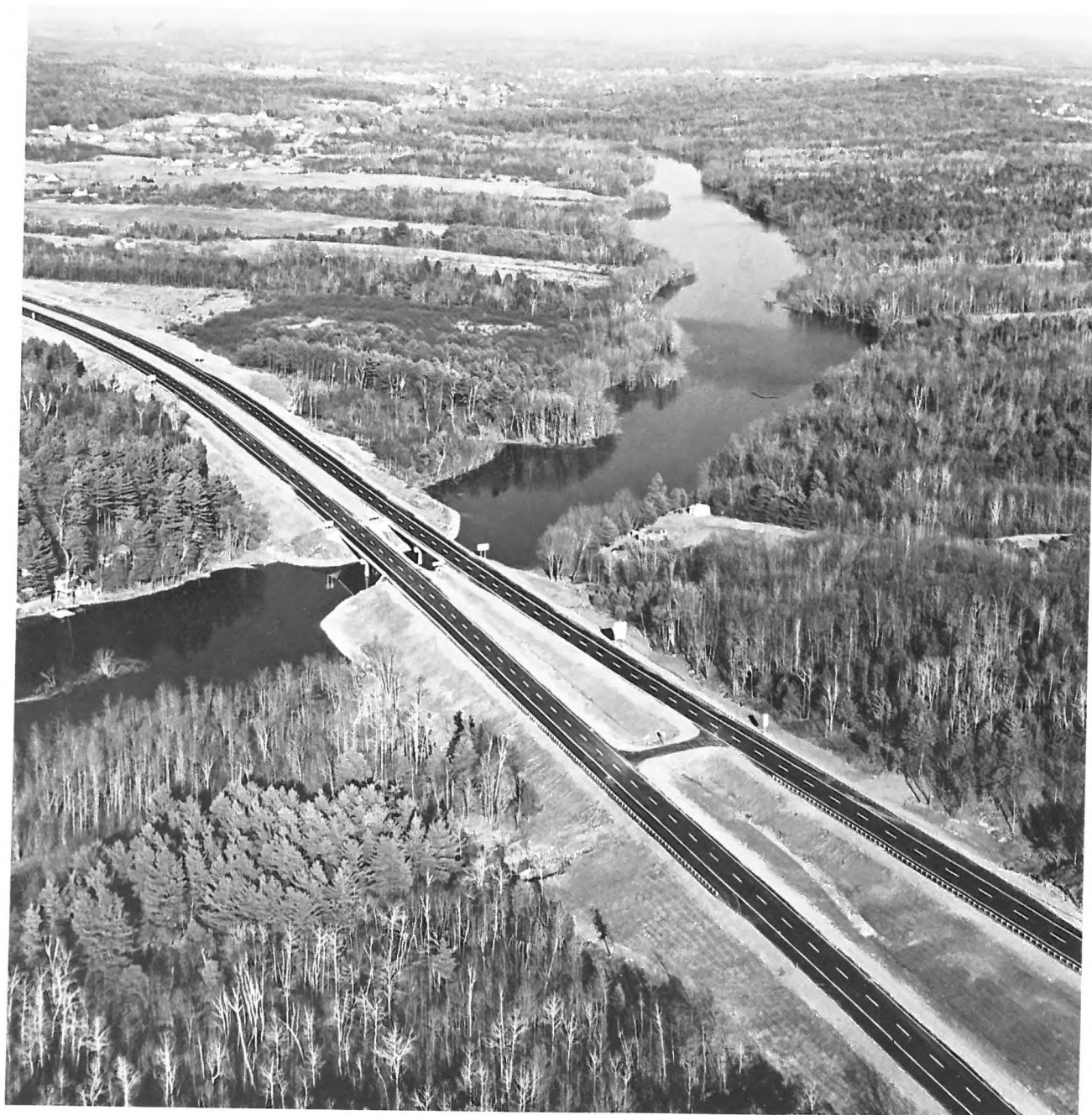
New section of I-95 crosses Cobbosseecontee Stream in Gardiner.
