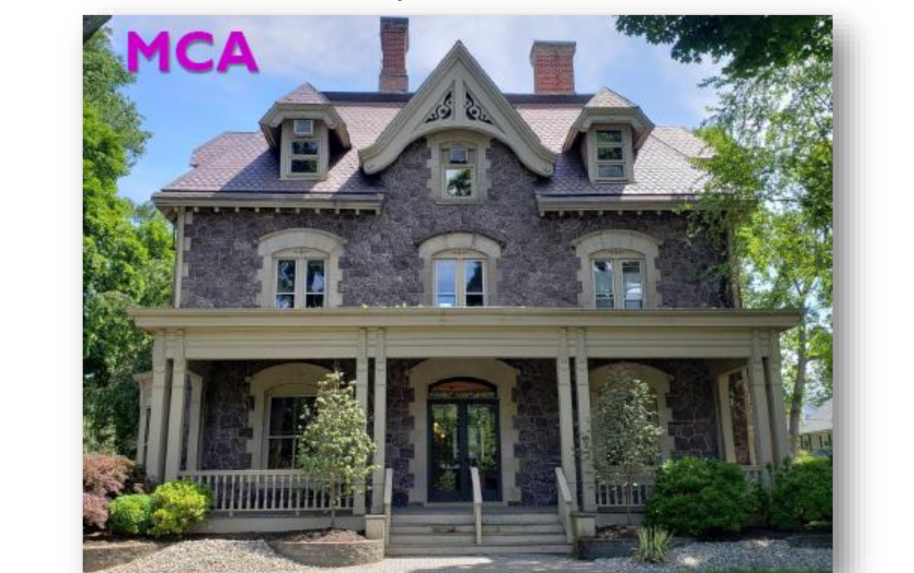
MCA Figure 10, MCA = 66 MacCulloch Avenue, Morristown. Built 1896. Faced with GPC veneer. Now offices. 6800 sq. ft.
