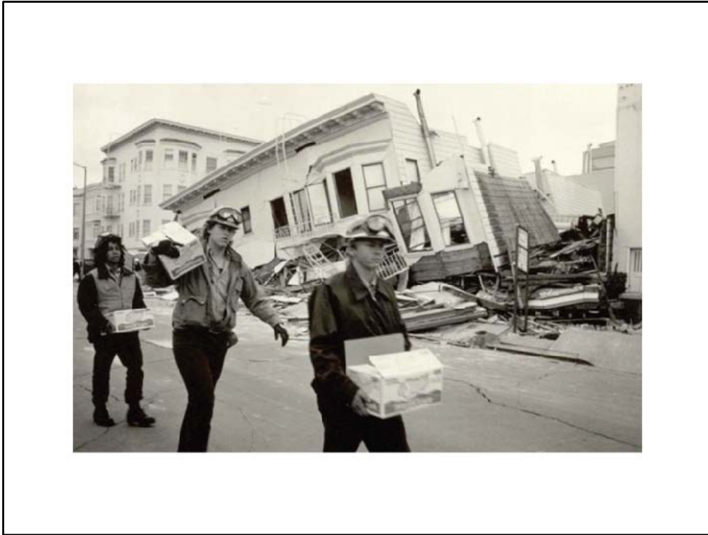
Figure 9. Aid workers carrying supplies past a collapsed building in San Francisco's Marina District in the aftermath of the 1989 Loma Prieta earthquake. Soils in the Marina District are prone to liquefaction (Fig. 8). (Photo: California Conservation Corps)
