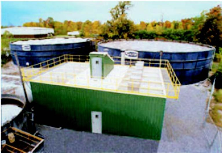
**Fig.6** Planta compacta UASB
