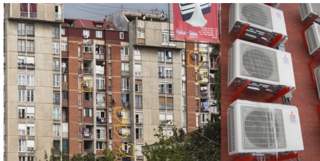
Photo of buildings in center of Prishtina. Circled are external air condition units
