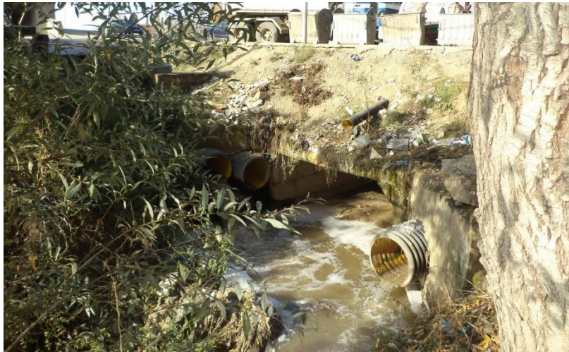
Discharge of domestic wastewater into the river Shtimjanka
