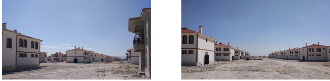
Figure 9. General views inside the construction site of Bozkır Barrage Resettlement Project (Süheyla Büyüksahin's personal archive, August 2020)
