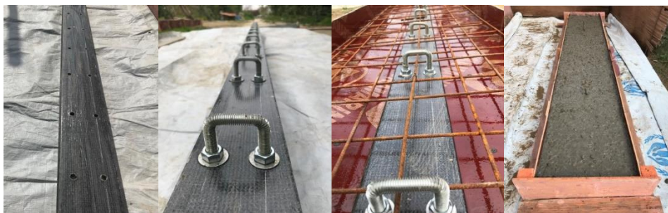
Figure 7. Preparation of the hybrid beam
