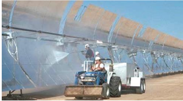
Figure 8. Manual cleaning of CSP mirrors using high-pressure spray [152].
