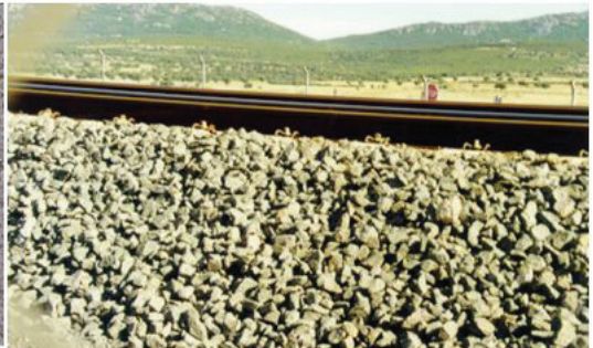
Figure 9. Basaltic ballast at the AVE railway.
