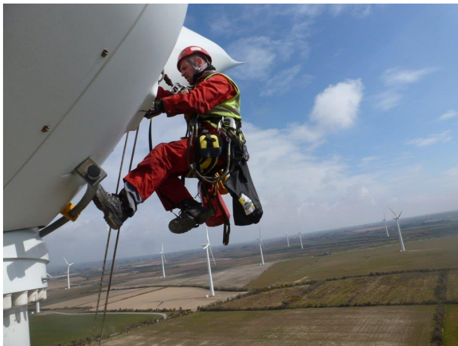
Figure 1. Maintenance technician making a repair labor in a wind turbine [15].
