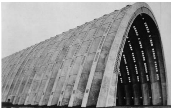
Figure 11. The two hangars are 175m long, 91m wide and 60m high. Connecting a series of parabolic arches formed an undulant vault similar to corrugated sheet, Orly (near Paris), France, Eugène Freyssinet, 1923. (Source of image: arquiscopio.com )
