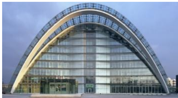
Figure 13. A parabolic two-hinged arch in Berliner Bogen Office Building, Hamburg, Germany, BRT Architekten. (Source of images: brt.de )
