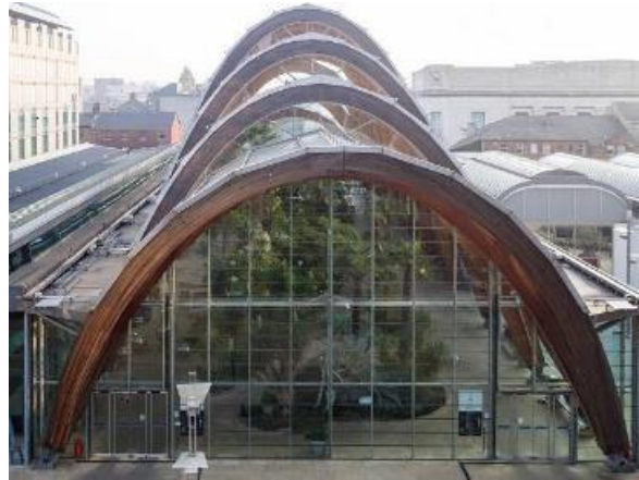
Figure 12. Glue-laminated two-hinged parabolic arches in winter garden, Sheffield, UK, Pringle Richard Sharrat Architects, 2002. (Source of images: prsarchitects.com and sheffieldnewsroom.co.uk )
