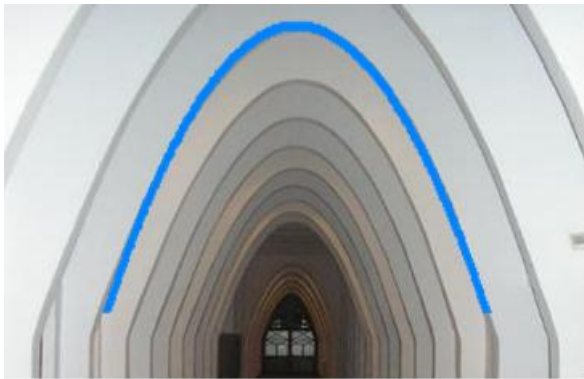
Figure 10. Parabola form on a set of repetitive parabolic arches in Colegio de las Teresianas, Barcelona, Spain, Antonio Gaudí 1890. (Source of image: touristeye.com )
