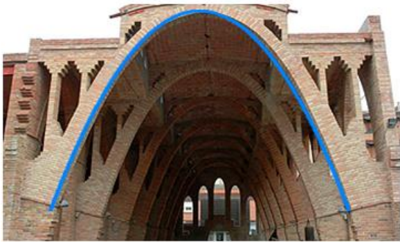
Figure 9. Masonry parabolic arch in Celler de Sant Cugat, Cèsar Martinell i Brunet, Spain, 1921. And form of the parabola (in blue) on it. (Source: http://patrimoni.gencat.cat )
