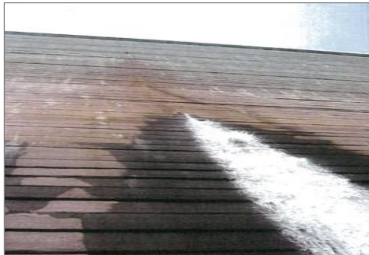
Figure 2.6 Cracks at Upper Stillwater dam (Smoak, 1991)
