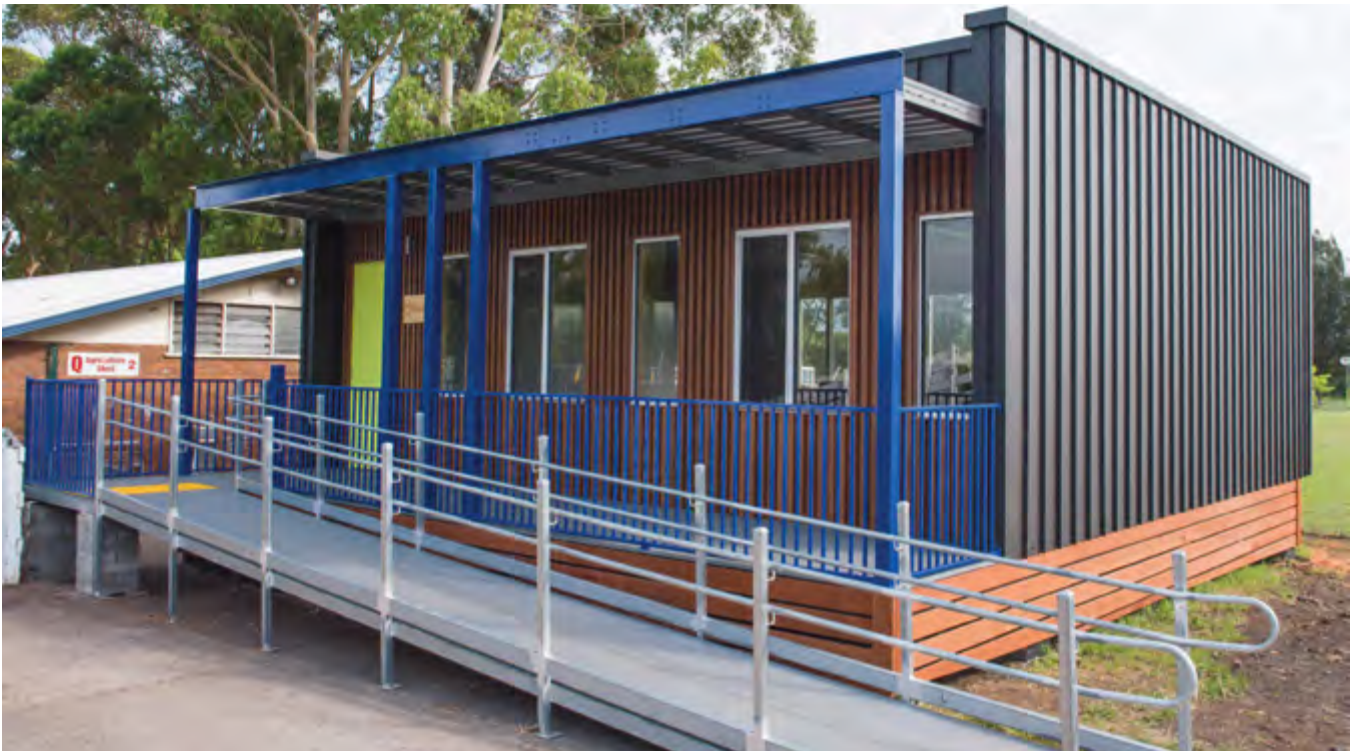
Figure 17: Modular classroom sample with solar powered roofs, thermal insulation in glazing and universal access. Source: https://hivve.com.au/news/
