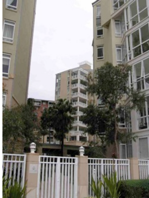
Plate8: New Fortified Harbourside Residential Areas A.P. 2004
