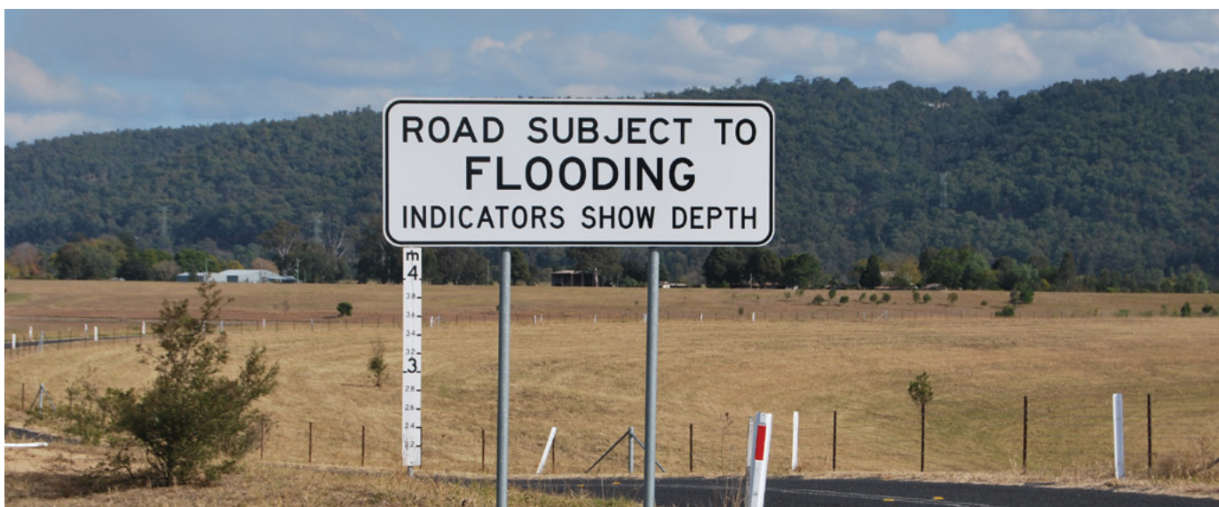
Roads in the floodplain showing inundation levels – sign (Western Sydney University)
