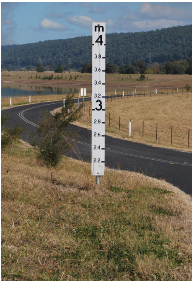
Roads in floodplain showing height of potential flooding (Western Sydney University)
