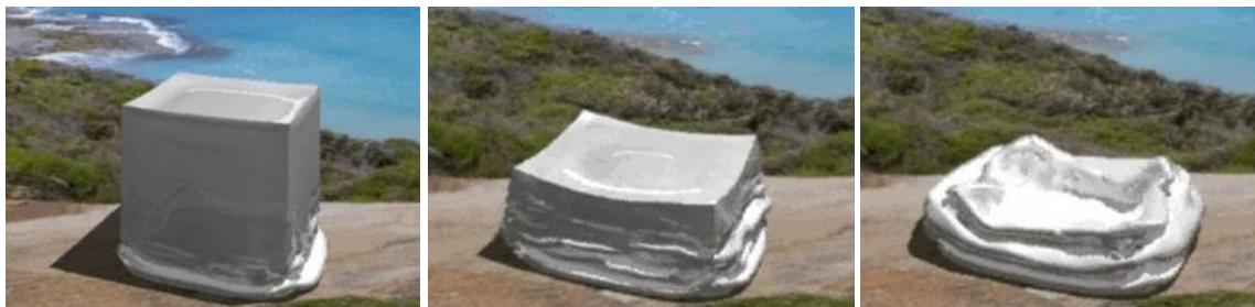
Figure 10.1: Pneumatic formwork installation steps of introduced system
