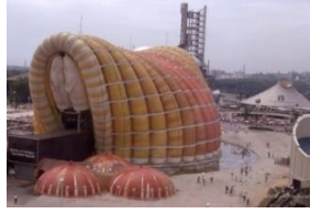
Figure 1.9: The Fuji Pavilion, an example for structural application of air-inflated rib structures [19]
