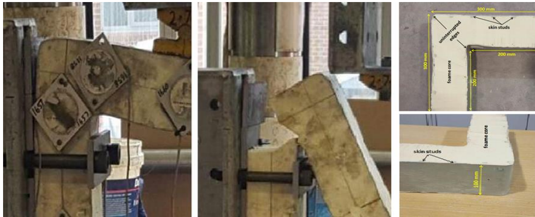
Figure 2.10: The ultimate deflection and the mechanism of collapse and dimensions of the connection
