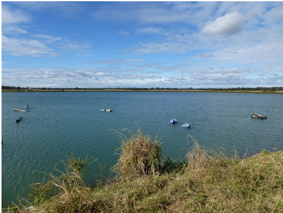
Figure 3.7 Turkey nest dam to store recycled water in HWRS
