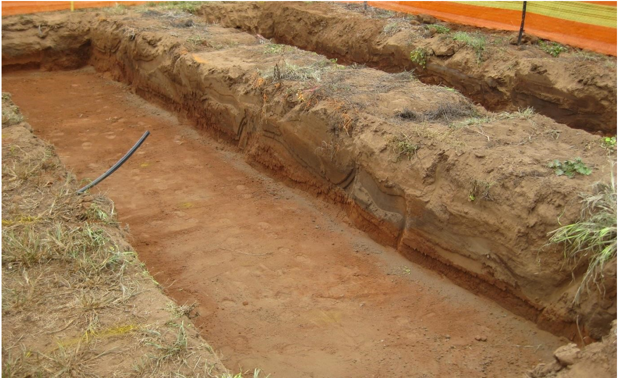
Figure A.3: Trench preparations for the field experiment
