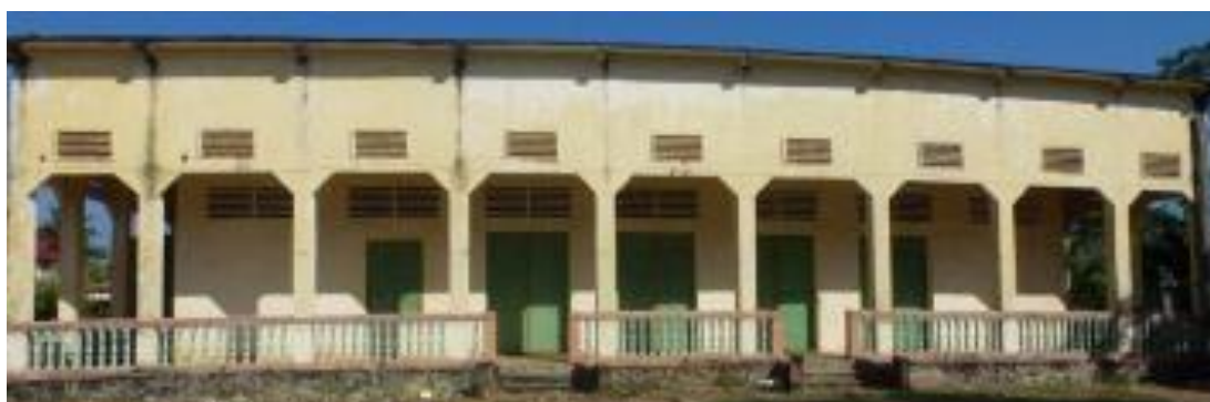
Figure 52: Building at Wat Nokor Bachaey, made available for the bamboo furniture workshop
