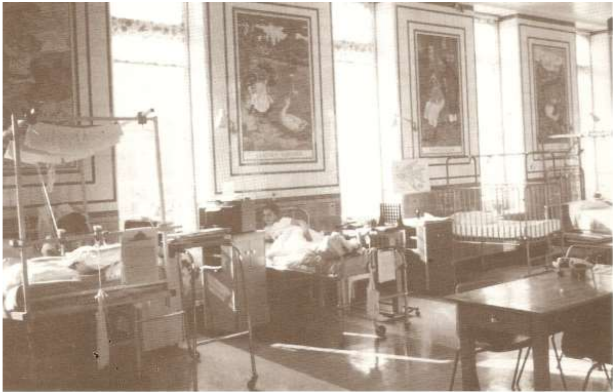
Figure 4-2 Victorian Children's Ward , this photograph show how the tiles were designed to fit neatly between the large windows of the pavilion hospital wards favoured by Nightingale and her contemporaries. Source John Greene's, Brightening the Long Days: Hospital Tile Pictures .
