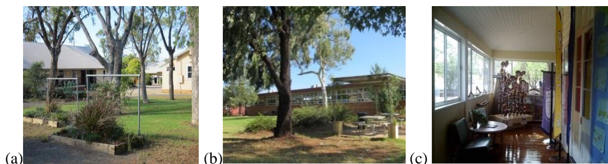
Figure 6.2 (a) 'Portable' primary buildings at Parkeview Central among native gardens, and; (b) secondary technology buildings, and; (c) Aboriginal artefacts and memorabilia in the administrative area
