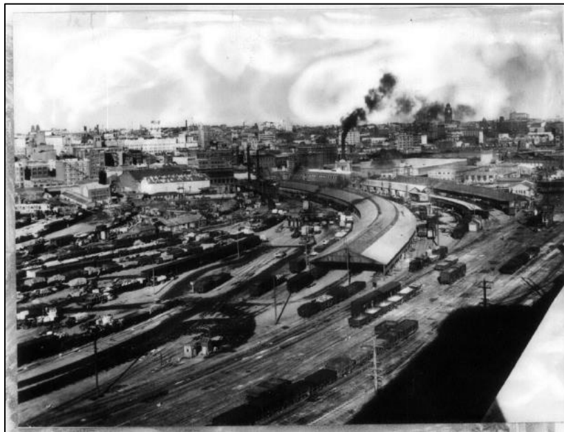
Fig 7.18: The Railway Goods Yard in 1946, showing the layout and the travelling gantry crane
