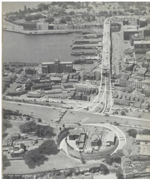
Fig 3.3: An aerial view of the construction of the Cahill Expressway in 1957, looking east from the Bradfield Highway
